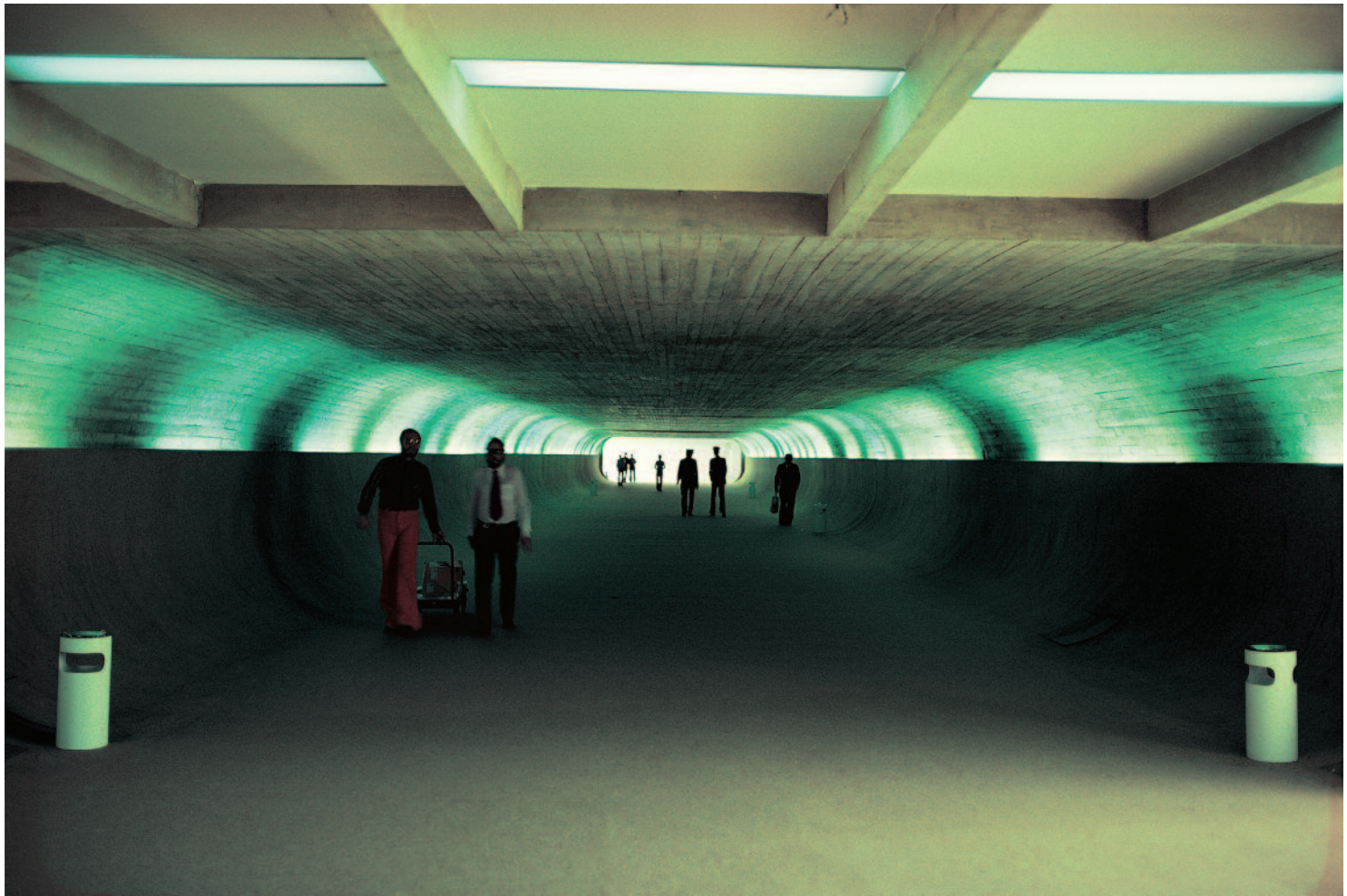
Underground corridor at the airport, Brasília, Brazil, 1977.
